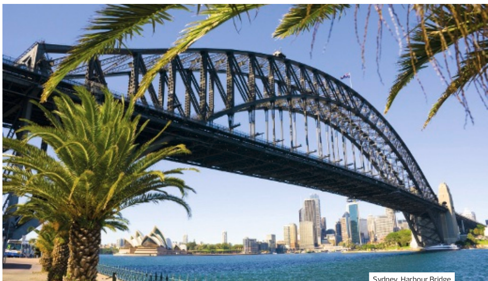
Sydney, Harbour Bridge
